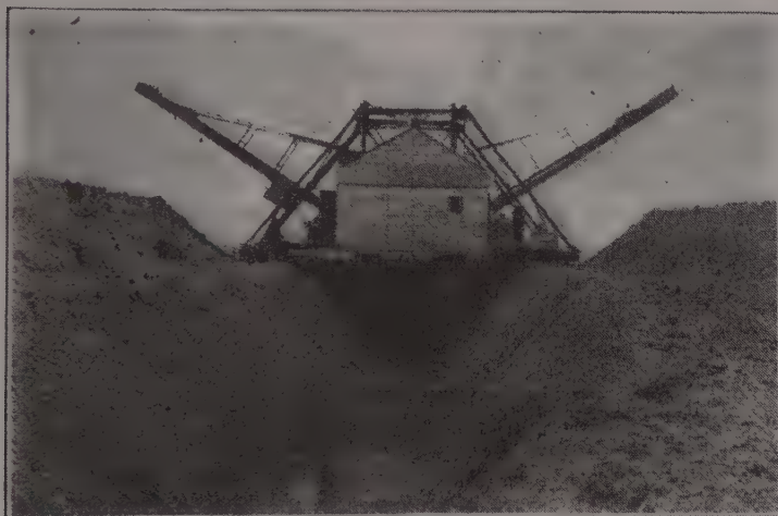
Fig. 67. An excavator for digging open ditches, which is carried on tracks laid at each side of the ditch.
