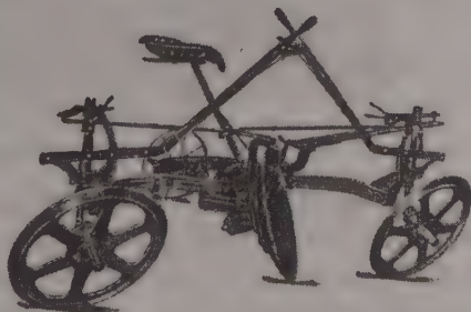
FIG. 117. A reversible disk plow. This plow is made to turn a right or left furrow by swinging the hitch from one end to the other.
