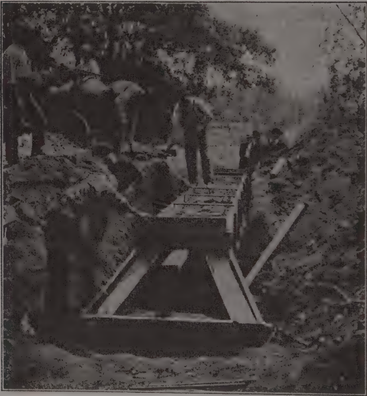
Fig. 95. Making a concrete culvert.
