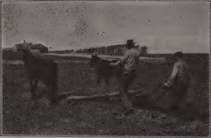
Fig. 61. Filling the ditch with a plow.
