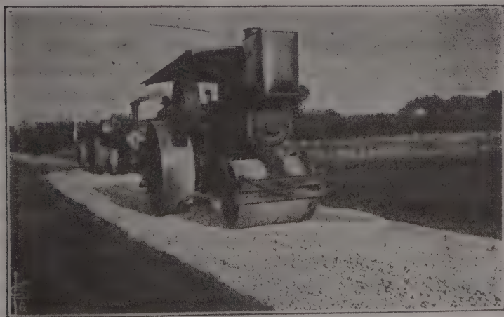
Fig. 84. Rolling the first course of stone.
