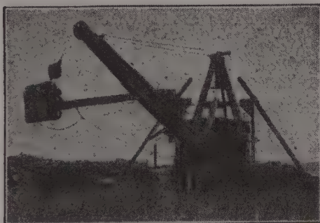
Fig. 66. A floating dredge for digging open ditches.
