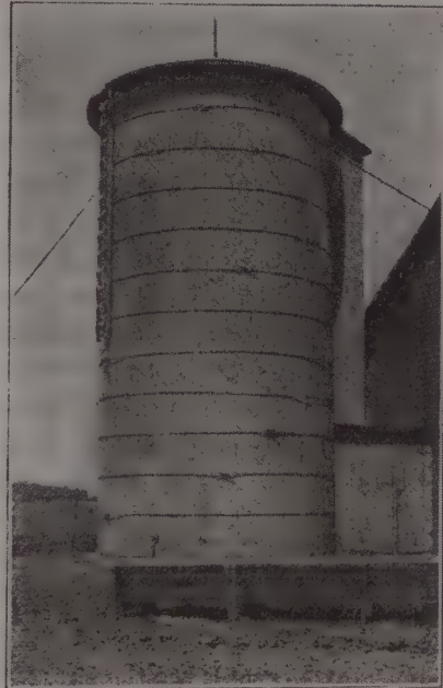
Fig. 294. A good stave silo well anchored.
