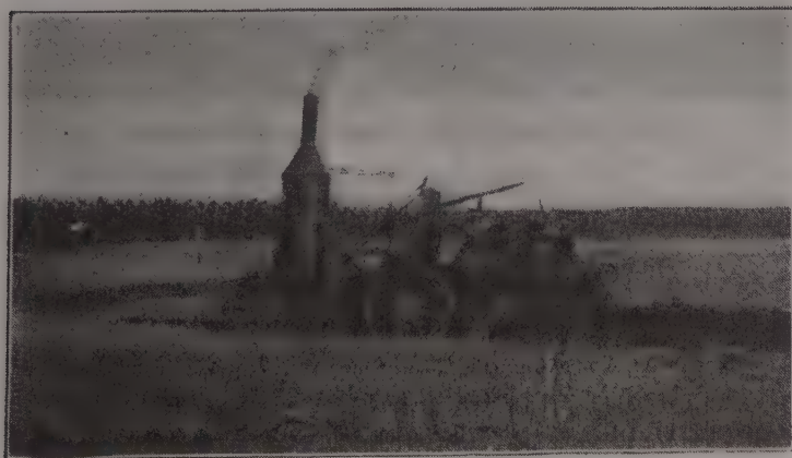
Fig. 54. A tile ditching machine at work.
