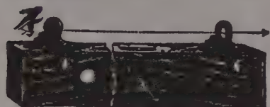
Fig. 23. A carpenter's level with sights attached.
