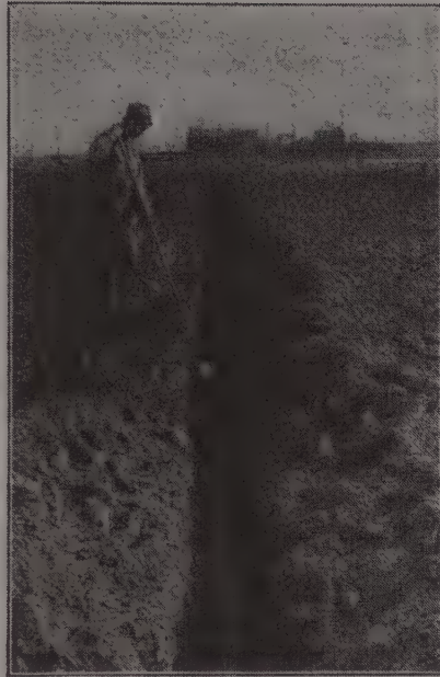
Fig. 59. Laying tile with the tile hook.
