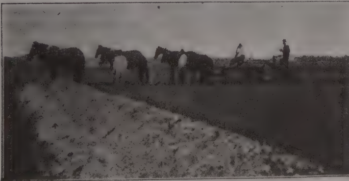
Fig. 62. Filling the ditch with a road grader.
