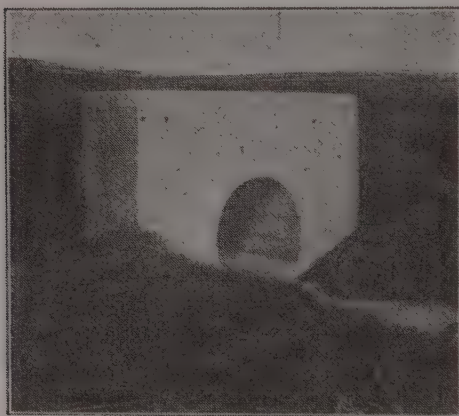
Fig. 63. A good outlet protection for a tile drain. It is desirable, however, that grating or bars be placed across the outlet to keep out small animals.
