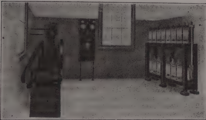
Fig. 318. Engine, dynamo, storage battery, and switchboard of an electric lighting plant.
