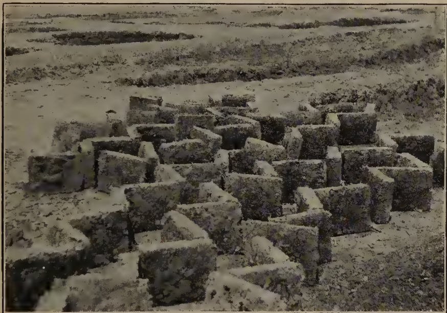
FIG. 74. -- Air-dried earth brick for house building.
