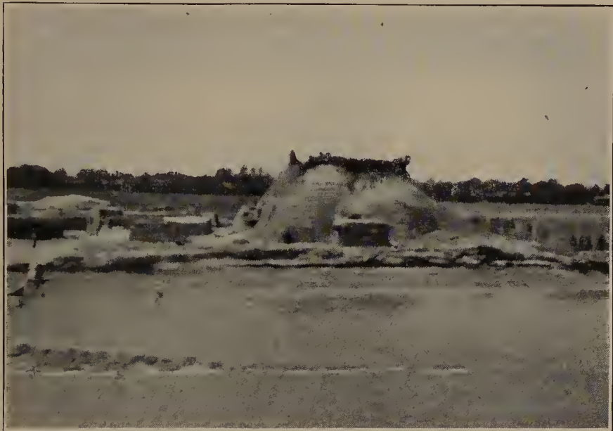
FIG. 76. — Earth and clay brick kiln on the bank of the Pei-ho, using sorghum stems for fuel.
