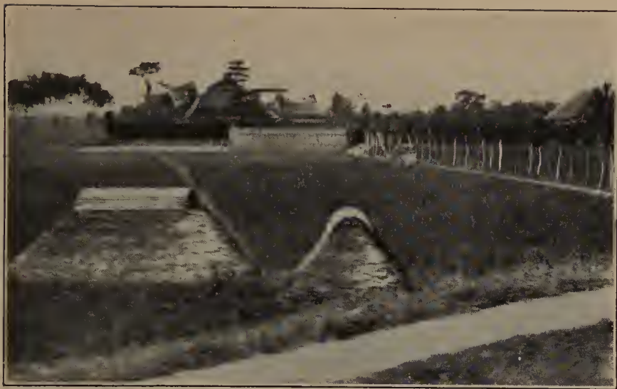
FIG. 94. - Japanese sheltered cement-lined storage pits for liquid manure.
