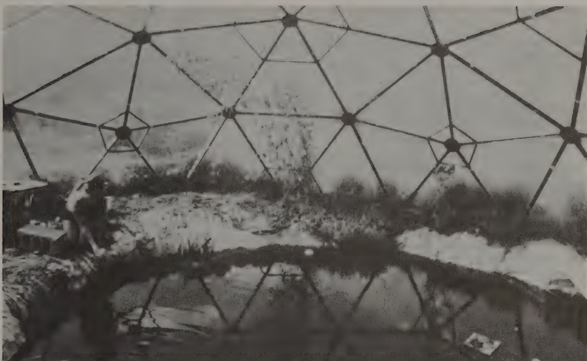
Backyard fish-farm greenhouse. Plastic above (double-walled Kalwall) holds heat in. Plastic below holds water in. The water circulates through a cohog-shell and bacteria natural filter which removes the chemical signals by which the fish population would normally stunt its own growth.
